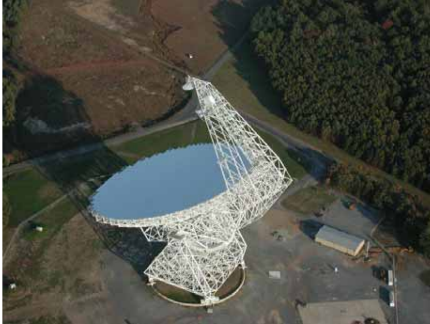
Figure 2-7: Green Bank Telescope (GBT): The largest fully steerable single dish in the world, 100 x 110 m. Located in Green Bank, Virginia, USA (c) National Radio Astronomy Observatory / Associated Universities, Inc. / National Science Foundation
